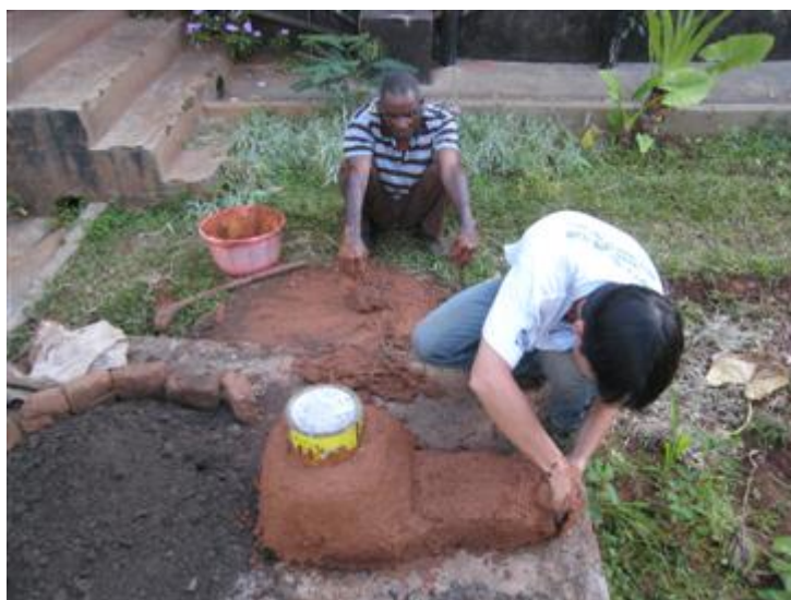
Learning by doing: Constructing a firewood saving stove in my own back yard
